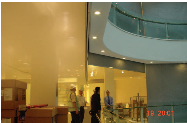
Smoke curtains being lowered in a major department store (left and below)
