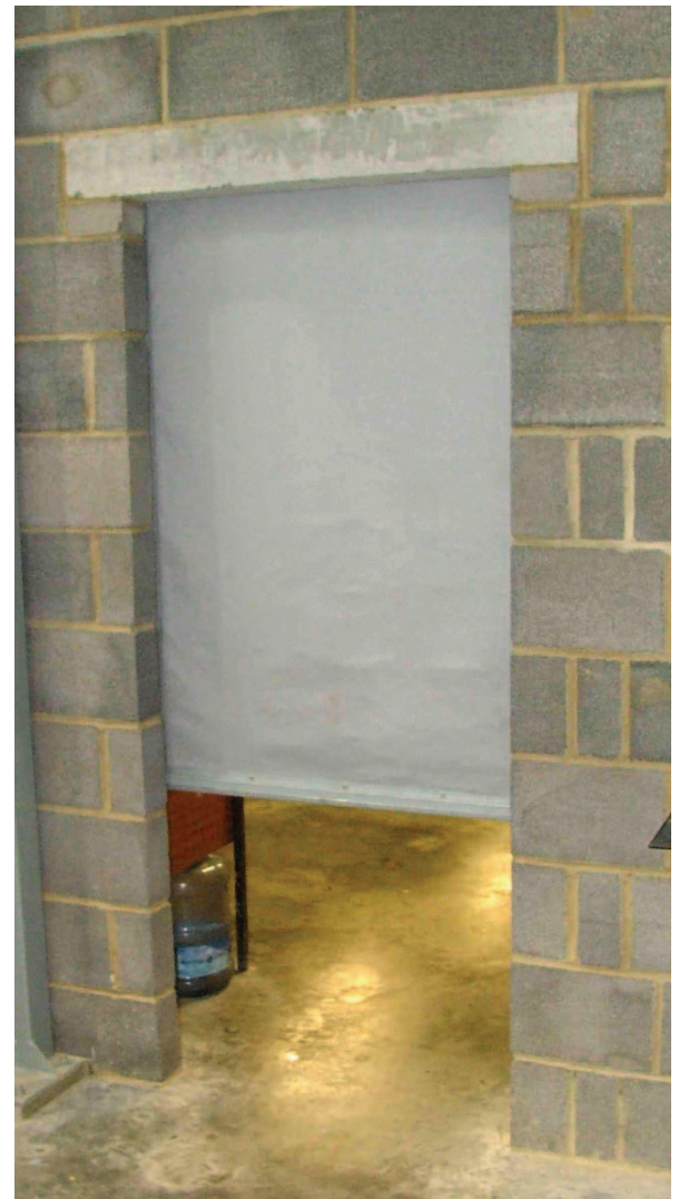
Smoke curtain provides virtual fire door for small to medium size opening in fire compartment wall
